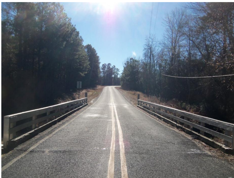
Photograph No. 2: This photograph was taken from the North Approach of the -L- alignment, looking South
