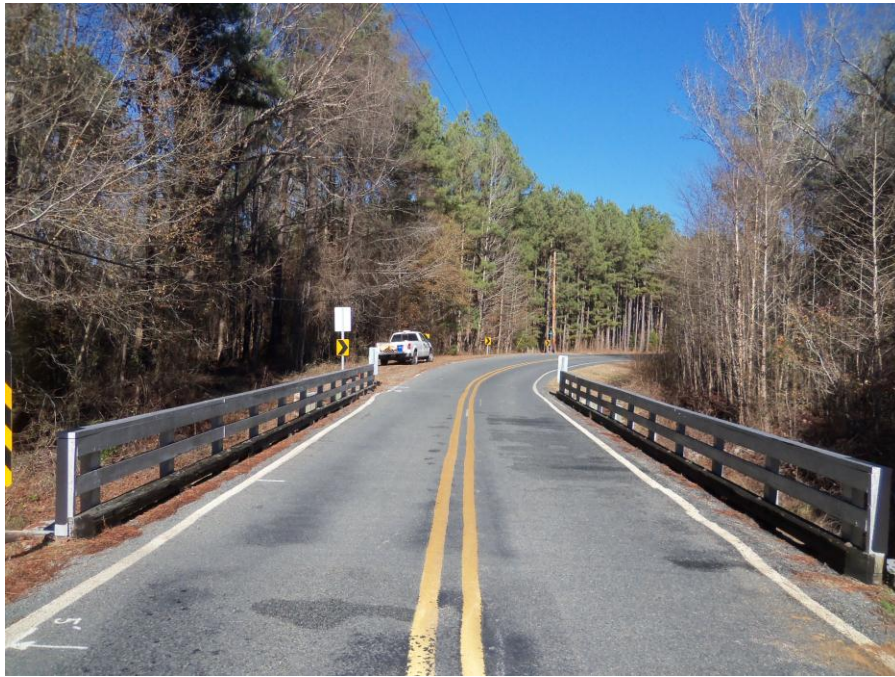
Photograph No. 1: This photograph was taken from the South approach of the -L- alignment, looking North
